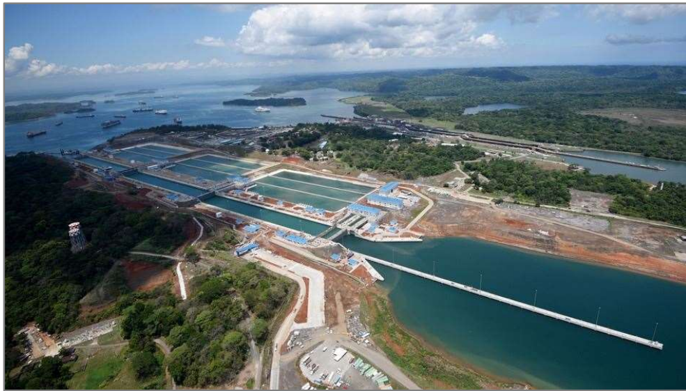
The New Agua Clara locks on the Panama Canal
