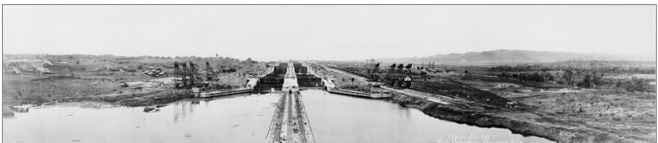
Construction of locks on the Panama Canal (1913)
