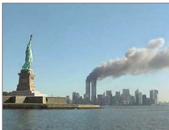
The Twin Towers of the World Trade Center burning before they collapsed on September 11 National Park Service
