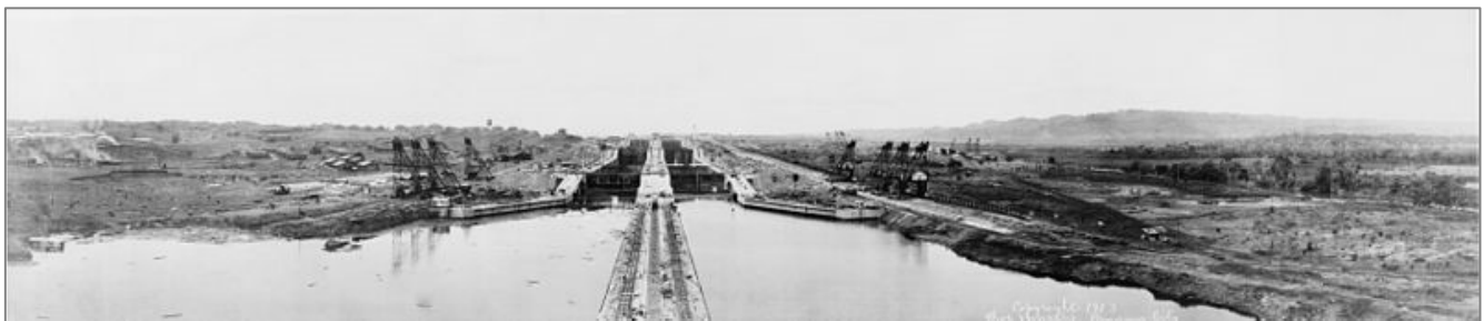
Construction of locks on the Panama Canal (1913)
