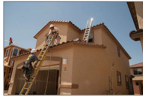
A residential construction site using fall arrest systems
