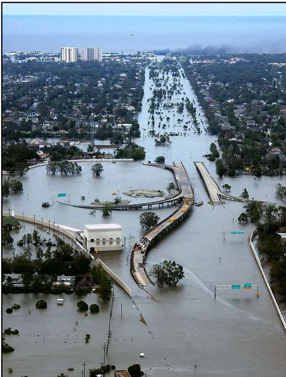
Flooded I-10/I-610/West End Blvd interchange and surrounding area of northwest New Orleans and Metairie, Louisiana
