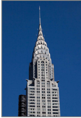
The Chrysler Building, considered the quintessential Art Deco skyscraper, located on the East side of Manhattan, New York City. Tony Hisgett from Birmingham, UK: Chrysler Building 1 , Uploaded by Magnus Manske. CC BY 2.0
