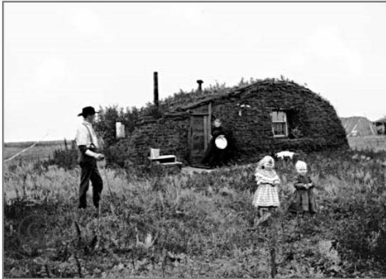
Norwegian settlers in 1898 North Dakota in front of their homestead, a sod hut
