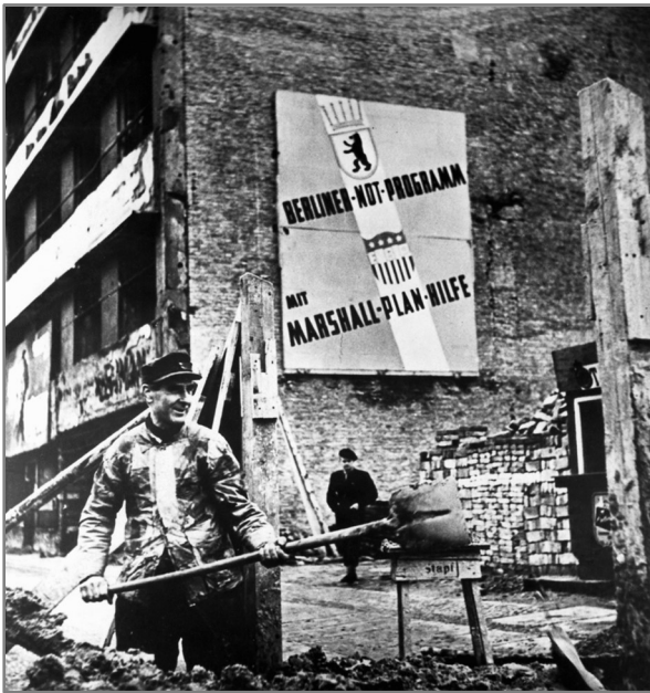
Construction in West Berlin with the help of the Marshall Plan after 1948. The plaque reads: "Emergency Program Berlin—with the help of the Marshall Plan."
