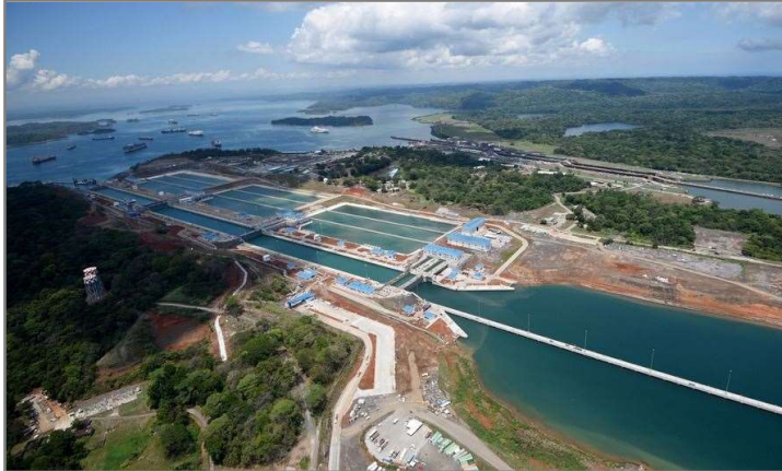
New Agua Clara locks (Atlantic side of the Panama Canal) in operation
